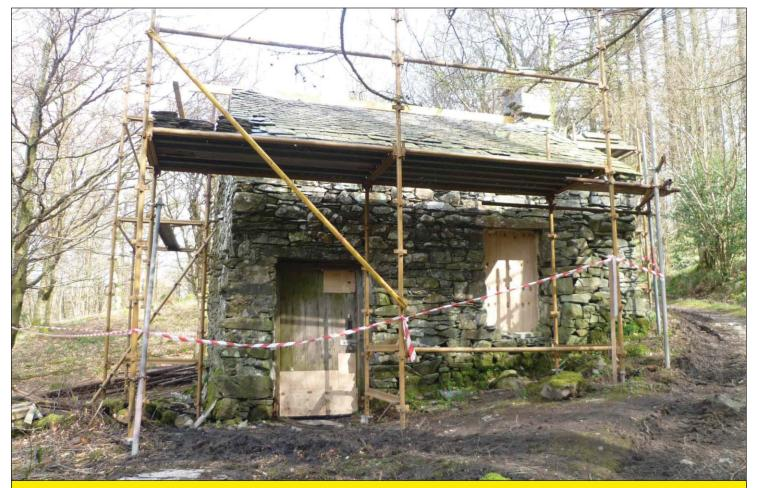
Mid-restoration. Scaffolding up and the roof about to come off for repairs to the timbers. Encroaching undergrowth cleared away
