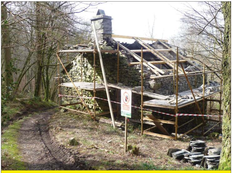
View from up the track showing the roof timbers in the process of replacement. Note 'elf 'n safety' signs and caution tape!
